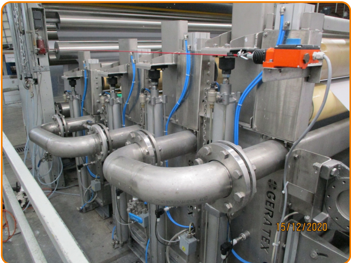
Geratex Scouring line installed in Germany
